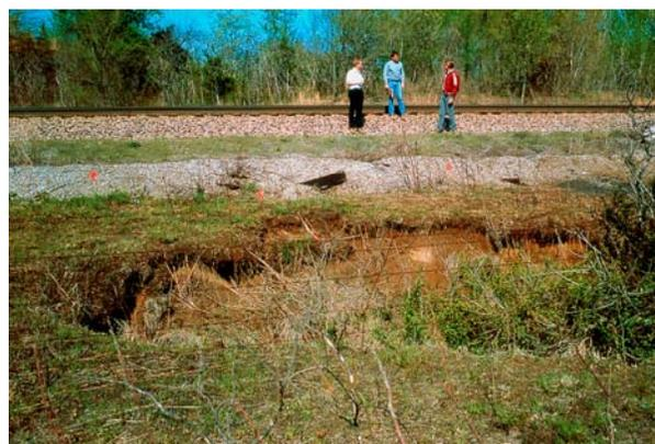
Figure 2. Mobilized soils from surface water cascading down an old vertical mine air vent.
